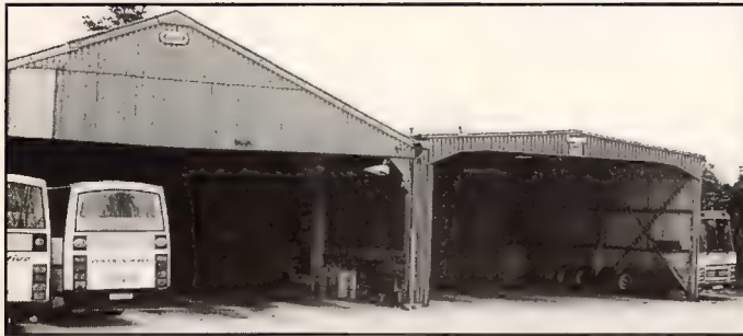
The depot buildings.
